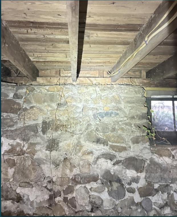
Basement Rim Joists/ Penetrations
