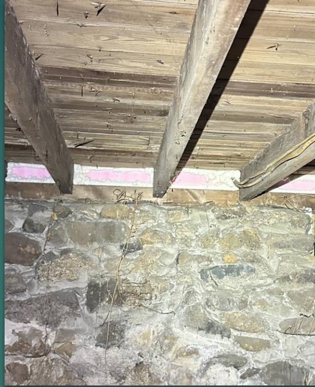
Basement Rim Joists/ Penetrations
